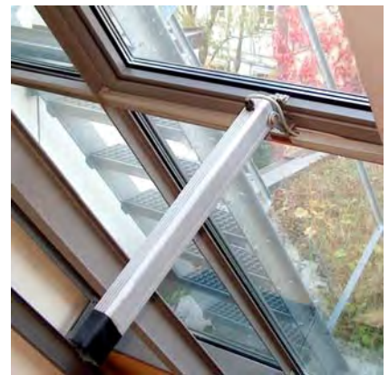
Example: facade area window Activation directly on HSK (Mounting on bar / waler)
